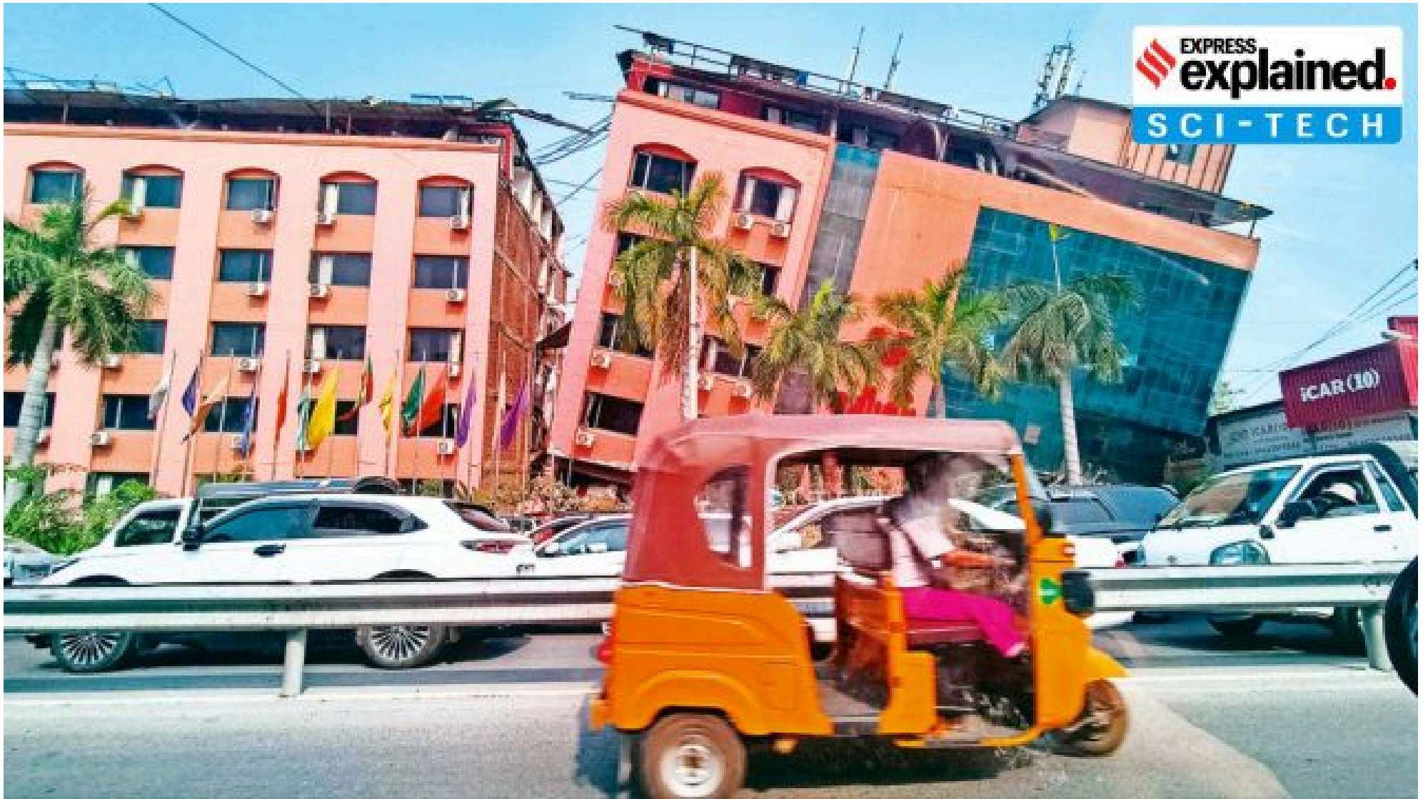
A damaged building in Mandalay, Myanmar, on Friday. (Reuters)
