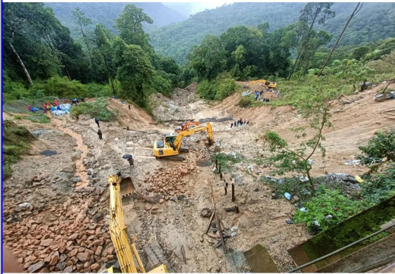
Personnel from the Mysuru Division of South Western Railway at work on the Hassan-Mangaluru line, near Kadagaravalli, Karnataka, on July 28, 2024. | Photo Credit: By Special Arrangement
