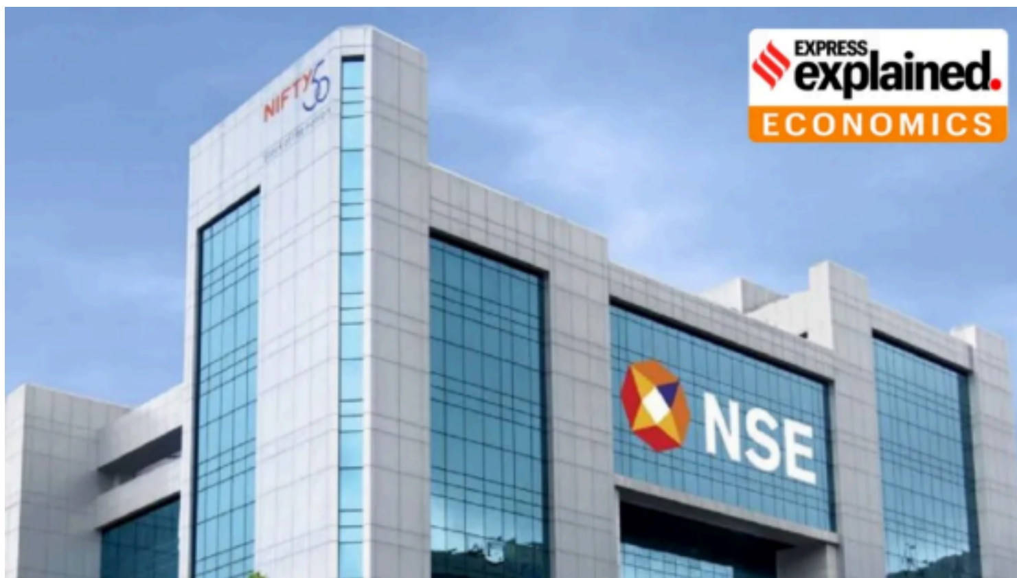
NSE Building (Wikimedia Commons)
